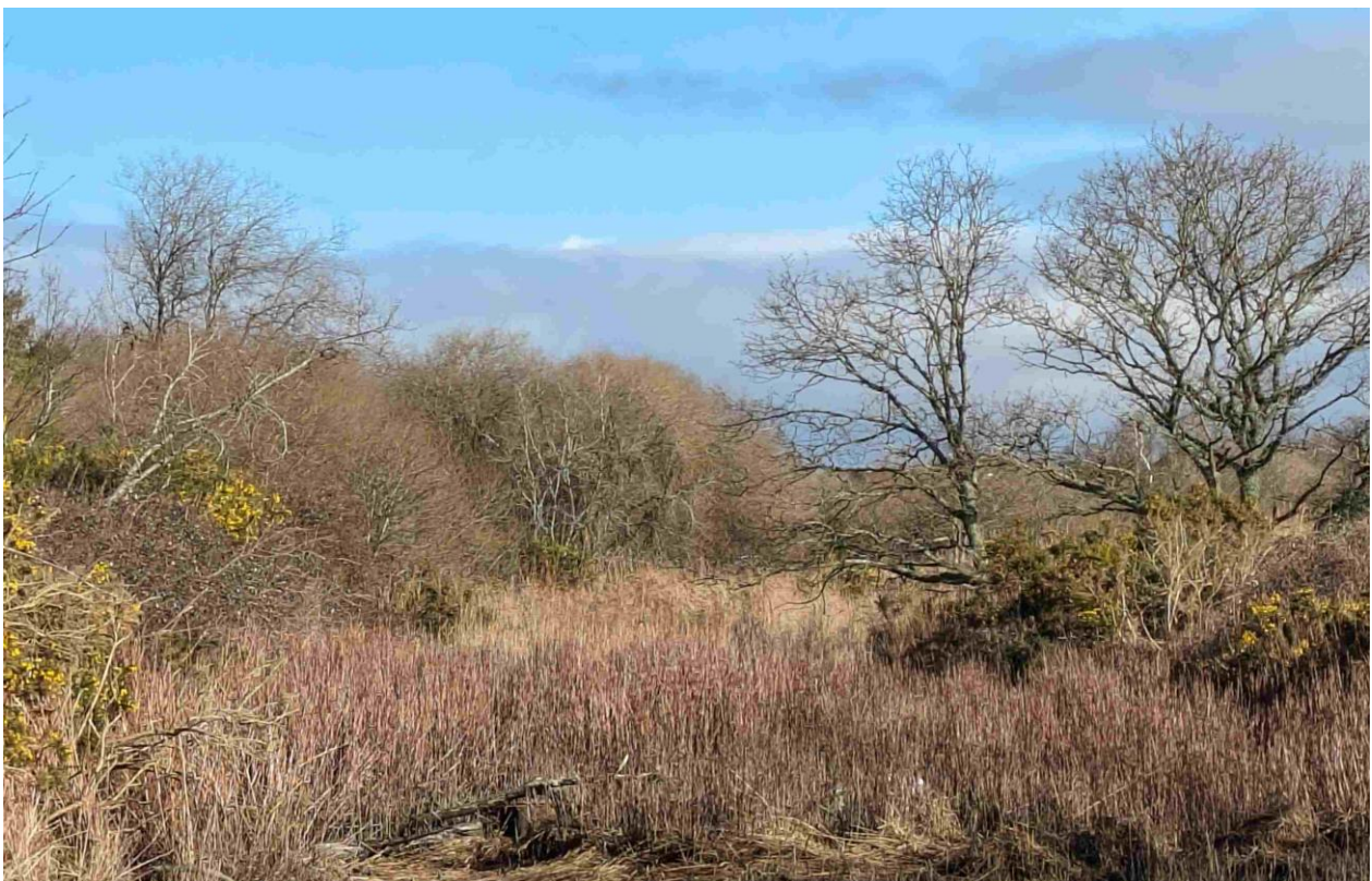
Today the outline of vertical sided cutting can still be made out even though they are now heavily vegetated. The bottom of the canal is soft mud filled with saltmarsh plants. © Shaun Robson
