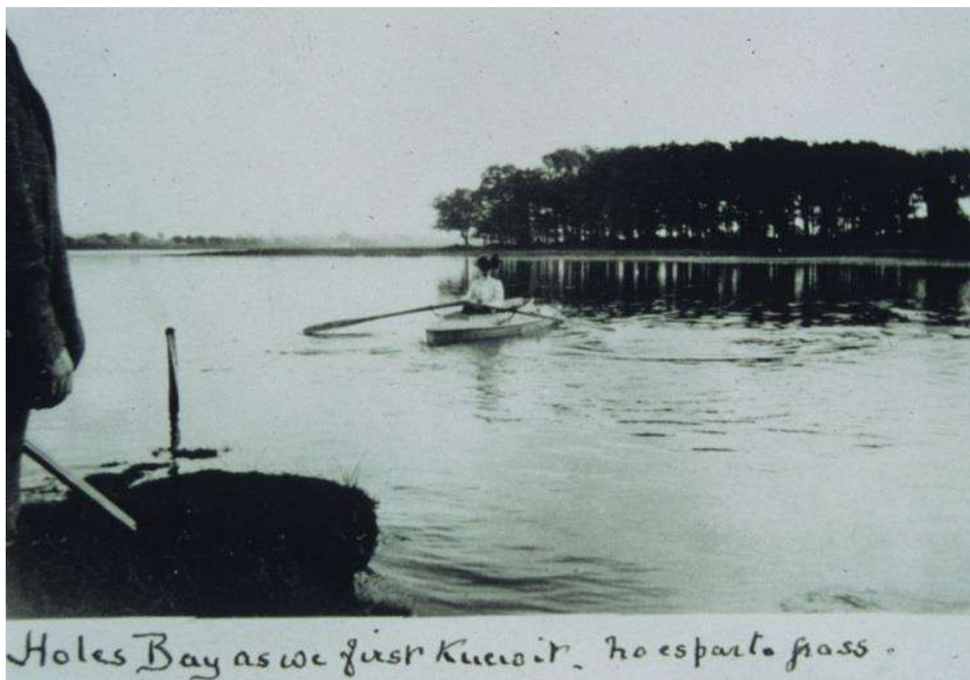
Fig 1 Llewelin family photo from the early twentieth century – “no esparto grass”.
